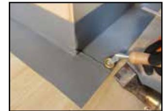
For perfectly sealed tape joints, weld the borders and press them together with the roller
