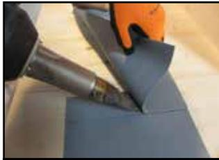
Heat tape surfaces using a hot air welding gun and press them together
