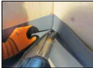
Heat tape surfaces using a hot air welding gun and press them together, starting from the corner working outwards
