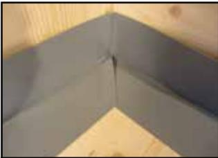
Cut to the centre of the tape and fit it into the internal corner; overlapping: > 2 cm, cut away the rest
