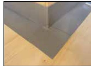
... fix it to the contact point in the corner also heated before; overlapping: > 2 cm
