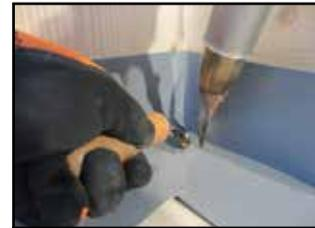
For perfectly sealed tape joints, weld the borders and press them together with the roller
