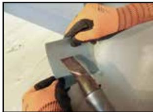
Cut a supplementary piece of tape; heat one corner using a hot air welding gun, stretch it slightly and ...
