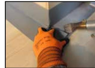
Heat tape surfaces and press them together, starting from the corner working outwards
